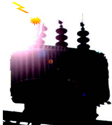
Gambar 6-60. Bushing trafo pecah
