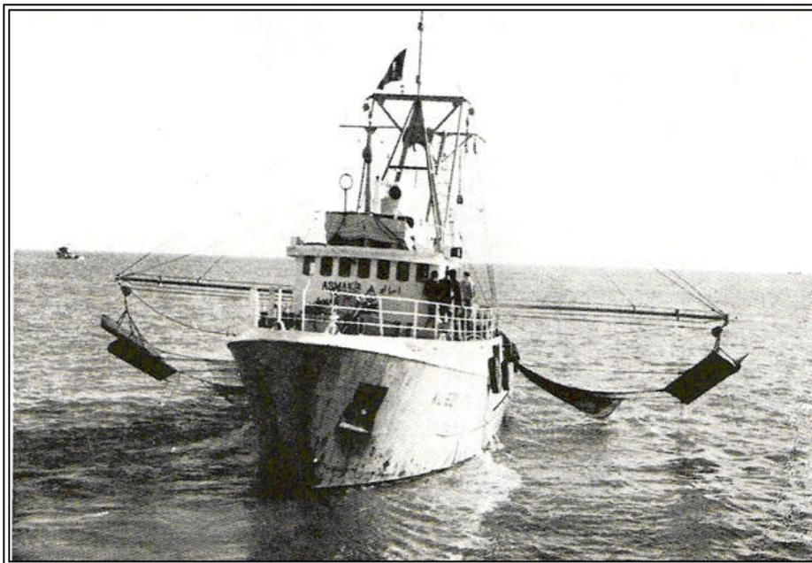
**Gambar. 14.8. Kapal penangkap *Double rigged trawl***
