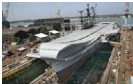
Gbr 4. 96dok kolom ( graving dock )
