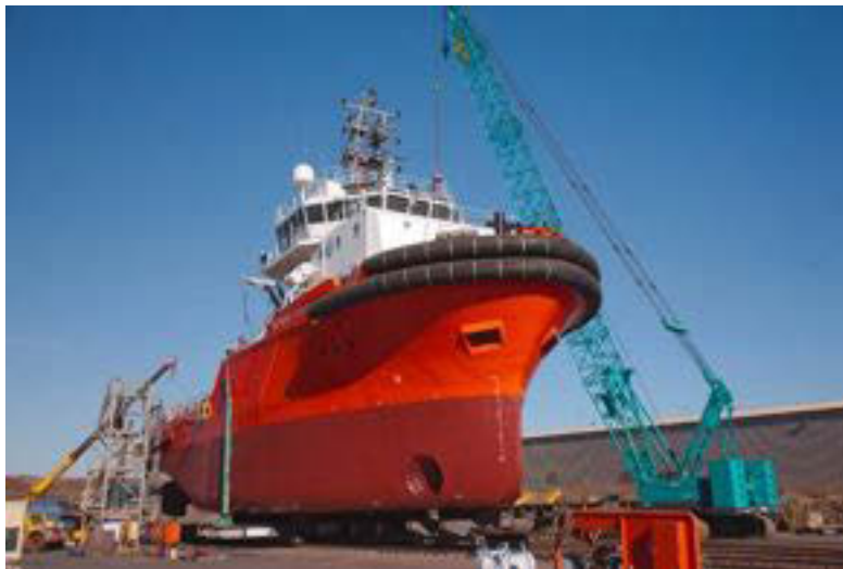
Gbr 4.82 Construction of Slipways to Dock the Vessels
