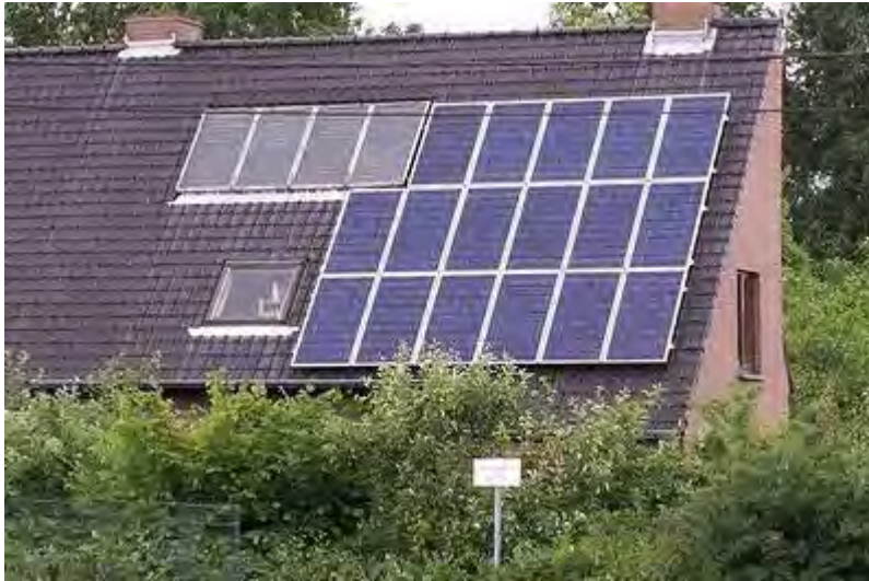
First Solar Inc,
