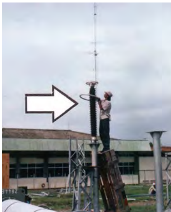
Gambar 3-5. Lightning Arrester (LA).
