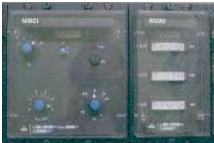
Gambar 3-19. Relay Differential Pilot Kabel.
